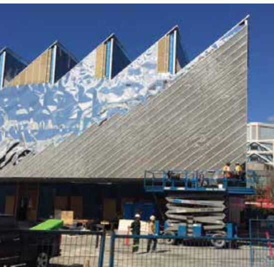
Install In Progress
