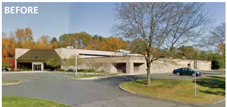
Structure prior to facade remodel
