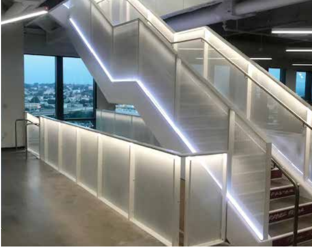
RAILING INFILL PANELS
