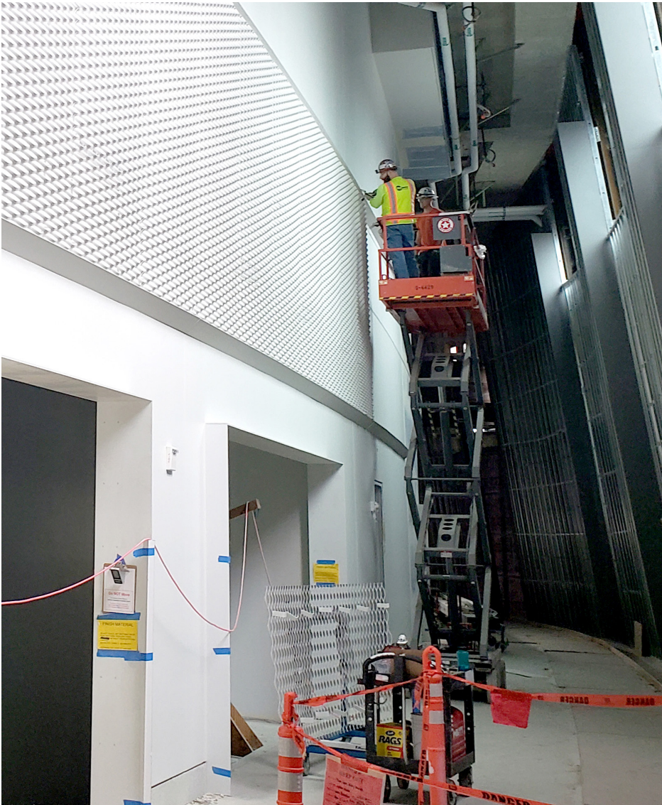
(LEFT) Shown is an in progress installation with an expanded mesh panel on the ground with brackets installed waiting to be lifted into place.
