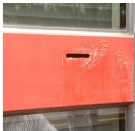
Figure 2. Filiform corrosion on Al (London 2013)
